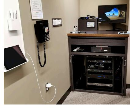
university's newest rooms, the eye lab, where an AT-UHD-CLSO-840 8x4 matrix switcher routes several inputs to three independent displays. A trio of AT-HDVS-200-TX-WP wall plate switchers connects to the CLSO-840 via HDBaseT. Each wall plate automatically selects between its HDMI and VGA inputs when a source is connected, and notifies the room's control system that a new device has been plugged in.
